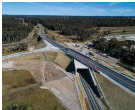
Rail access works.
