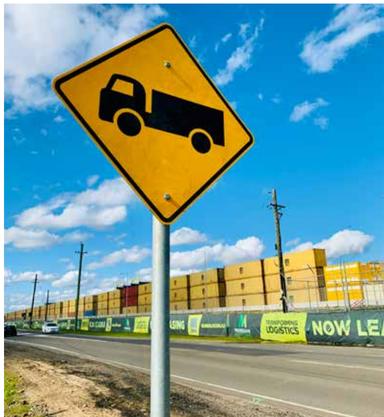
Moorebank Logistics Park is taking shape in Sydney's South West
